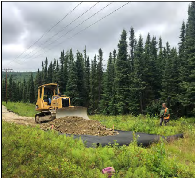
Constructing multi-use trail at Isberg Recreation Area. PHOTO: Bryant Wright
